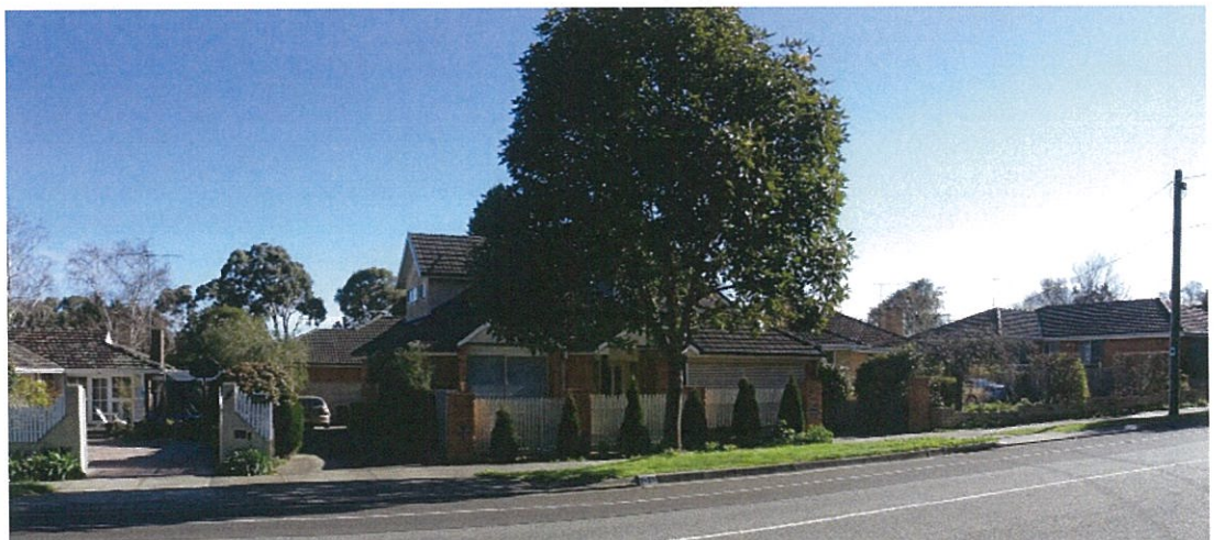
Figure 6: No. 33 Watsons Road, viewed from east side of Watsons Road
