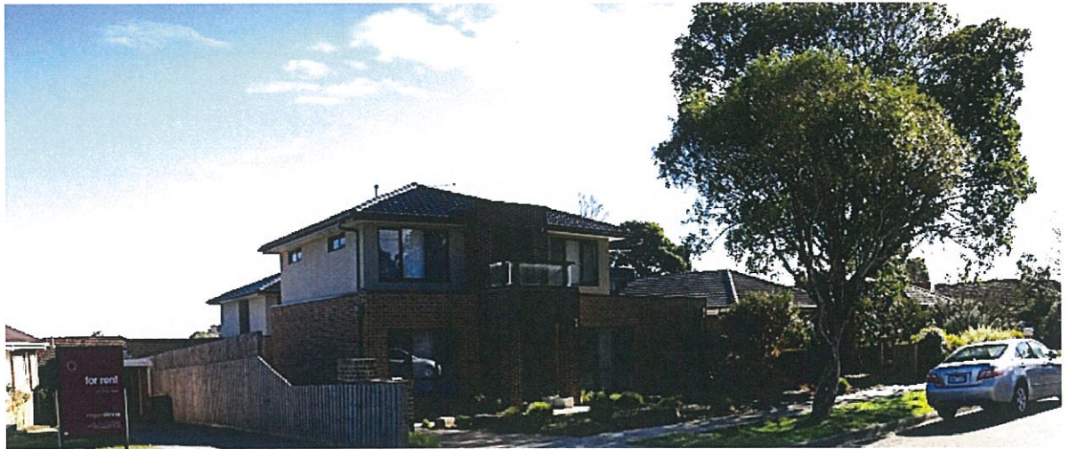
Figure 9: Two dwellings at No. 11 Dion Road, showing lightweight building materials on the second level.
