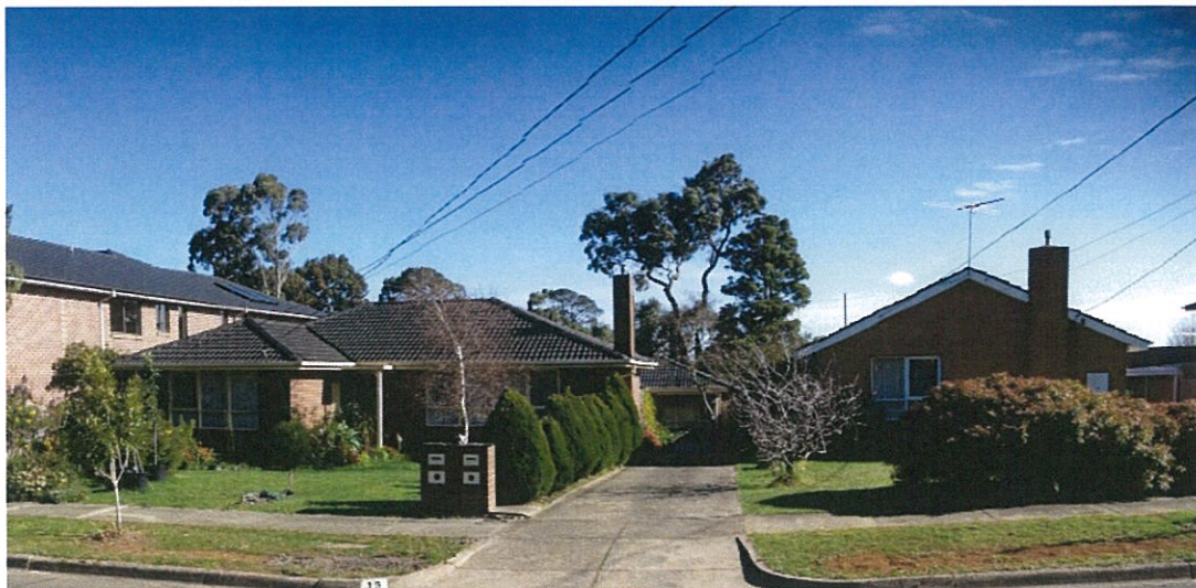
Figure 10: Two dwellings at No. 15 Dion Road
